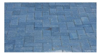
4"x8"x2-3/8" **Holland Stone Concrete Pavers** Stacking Pattern **PROPOSED**
